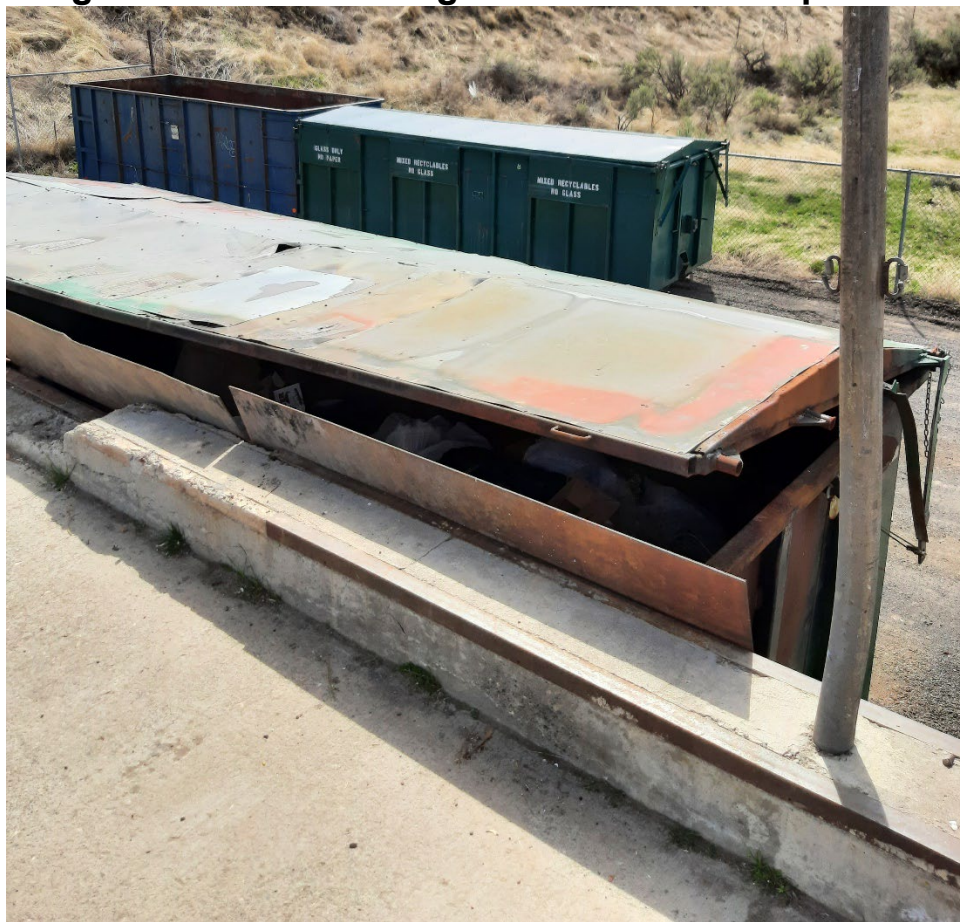
MSW tipping area
