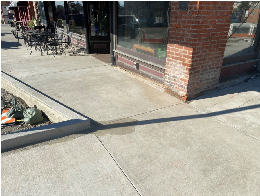
Figure 2: East ramp looking southwest
