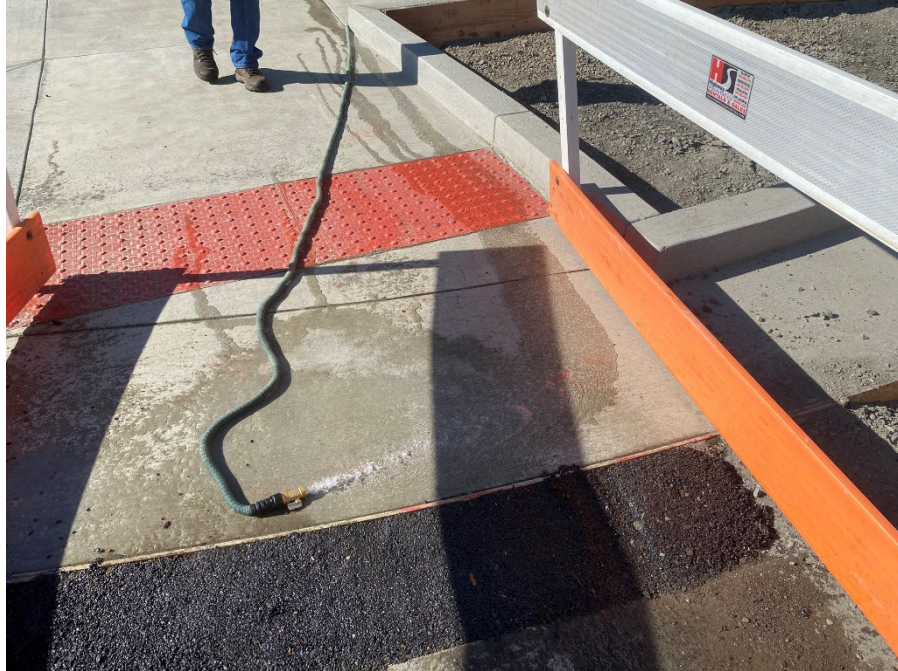
Figure 3: North ramp, looking south
