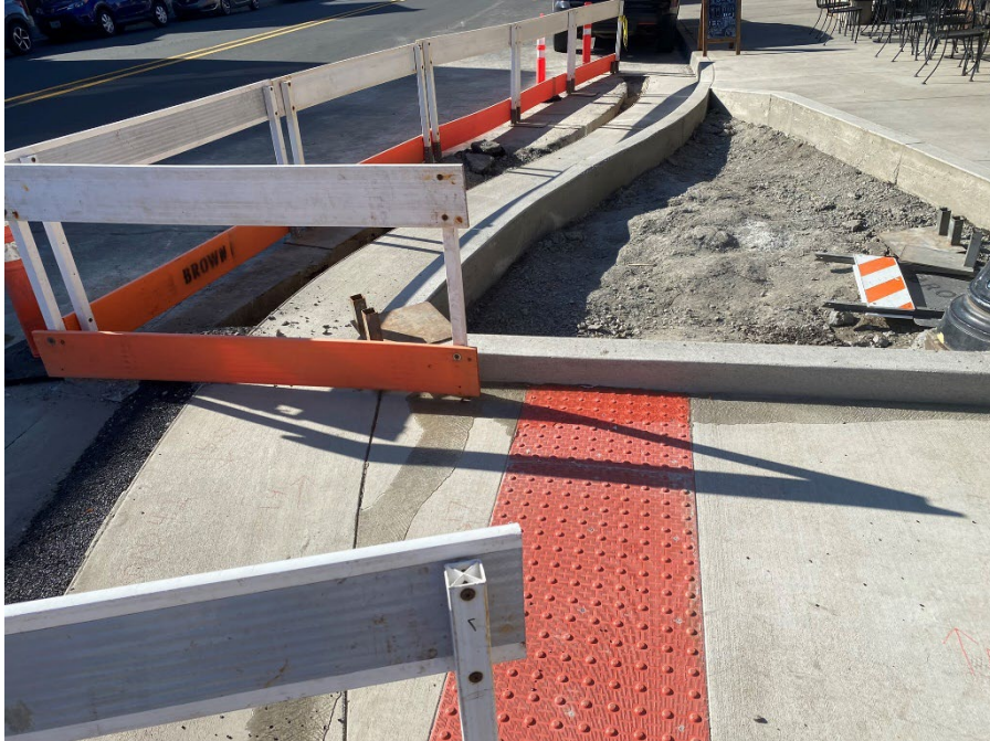
Figure 1: East ramp, looking southeast
