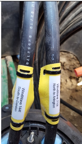
Figure 17. Transition from 144 Count Fiber to 216 Count Fiber
